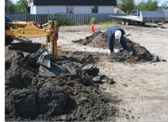
Soil testing (borehole)
