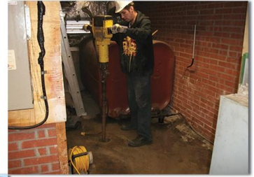
Soil testing (exploration trenches)
